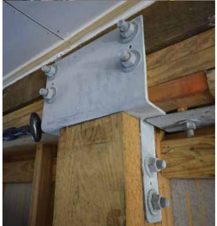
Top: Re-wiring masonry buildings after Hurricane Katrina. Bottom: Modern reinforcements between foundation and walls.
